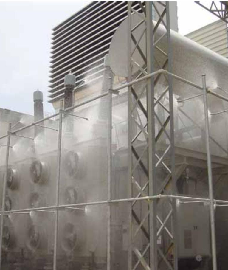
Minimax water spray systems are designed according to the individual needs of our customers and the fire protection requirements at the site, taking into account the actual fire load, structure of the building or the protected object. For special risks spray water fire extinguishing systems can be equipped also with foam proportioners for foam concentrates.
